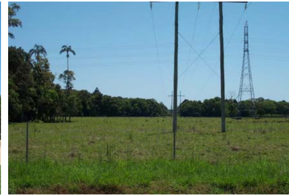
PN4 No vegetation under the powerline
