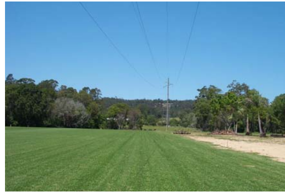
PN3 No vegetation under the powerline
